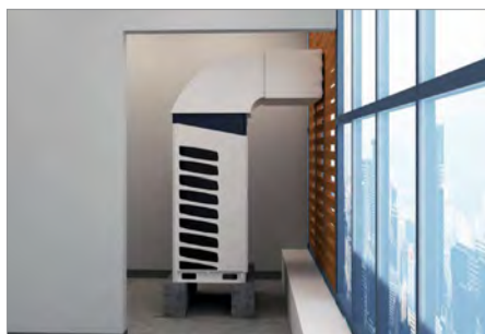
Installation of duct
